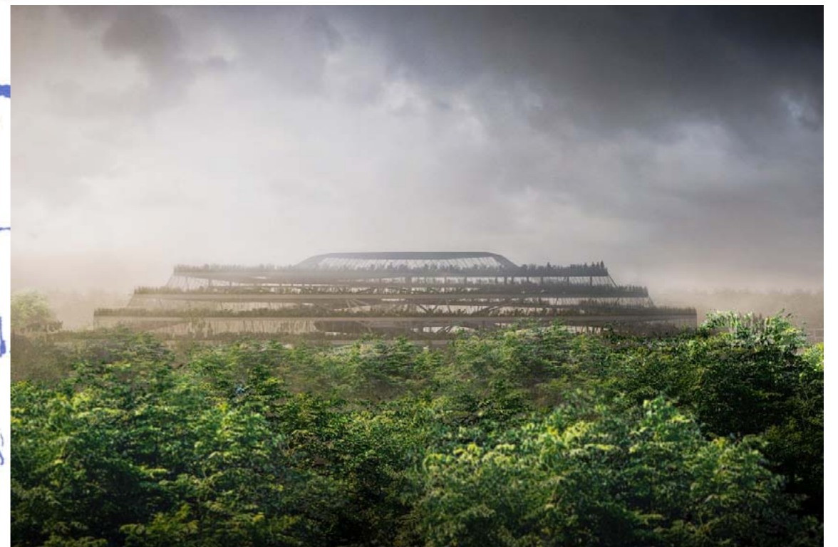
Water park AQUALAGON, Alain La Vallée, Jacques Ferrier Architectes pour Center Parks / Eurodisney SCA, 2015 (in progress)
